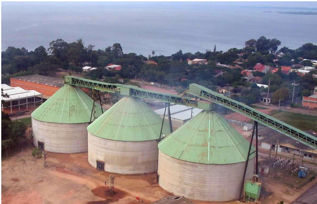
Chip silos for suitable wood mix control (Aracruz Celulose – Guaiba mill)
